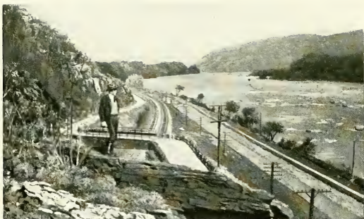
AN UNUSUAL SCENE—HIGHWAY, BALTIMORE AND OHIO TRACKS, C. & O. CANAL AND POTOMAC RIVER AT HARPER'S FERRY
